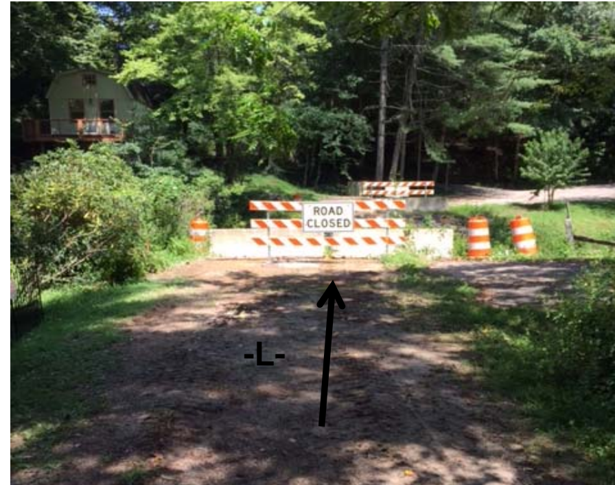
View looking east along proposed bridge alignment
